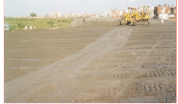
Construction of embankment with fly ash at Kalindi Bypass in Delhi
