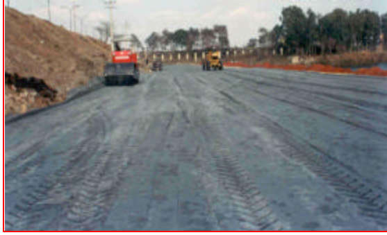
Construction of embankment with fly ash at Second Nizamuddin Bridge
