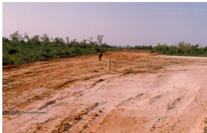
Jute geotextile treated section after cyclonic rains
