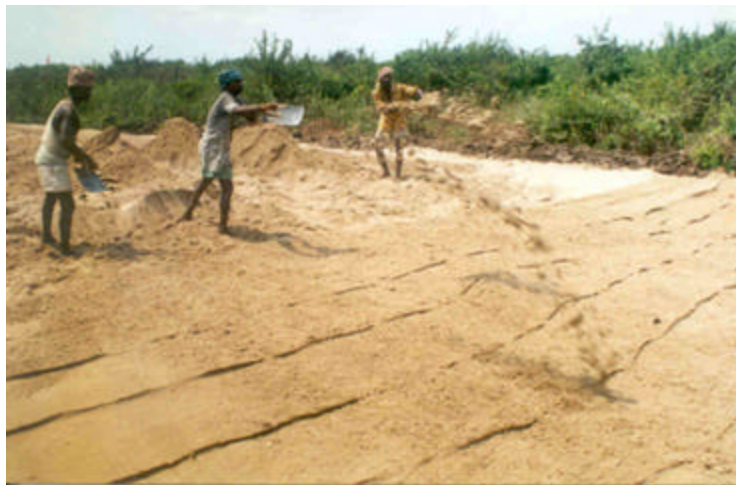
Laying of Jute Geotextiles for ground improvement
