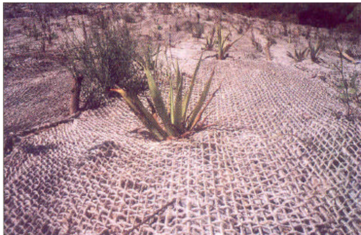
Growth of vegetation on slopes covered with jute geotextiles
