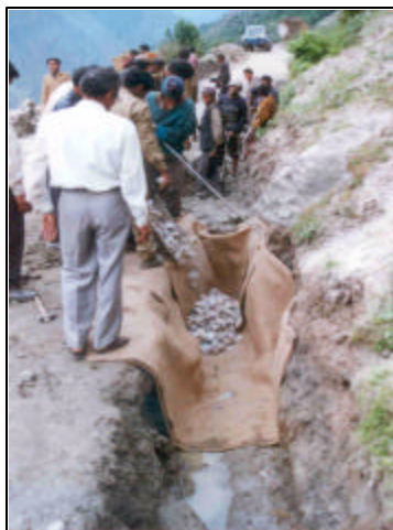
Laying of Jute geotextile as Trench Drain
