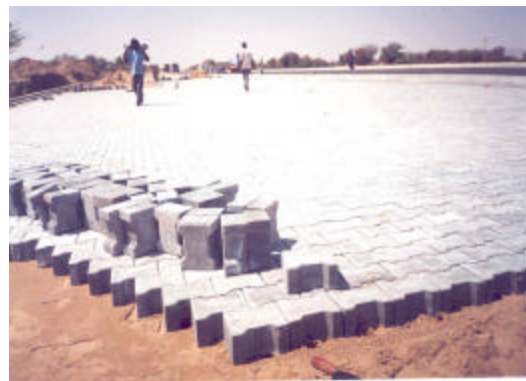
Photo –2: Laying of ICBP in Progress
