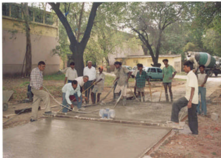
Fig.1: Construction of High Performance Concrete Pavements at CRRI Campus
