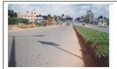
Photo 2 : View of road section with plastic after one year
