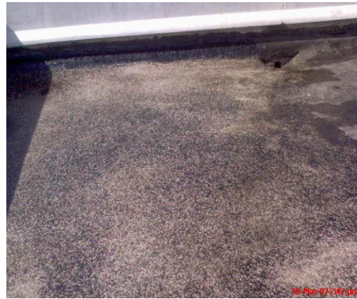
View of roof after water proofing treatment
