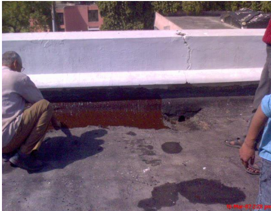
View of water proofing treatments
