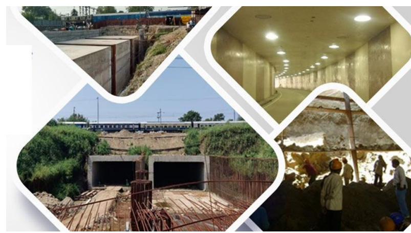
Stepwise repeated De-stabilisation and Stabilisation of collapsible soil mass by "Soil Nailing Technique" used for construction of Railway/Road underpass
