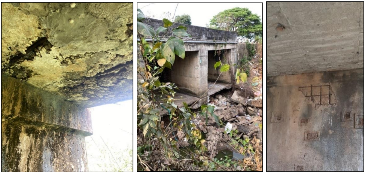
Figure 16: A Typical View of (a) Severely Exposed Reinforcement Observed on the Deck Slab of the Paiki Nallha Minor Bridge on Bhanjanagar- Tillisingi -Tarasingi Road at Ch. 29.550. (b) Erosion of the Apron of the Kotibaradi Bada Sankh Nallha Bridge on Bhanjanagar Tillisingi Tarasangi Daspalla Road at Ch. 9.580 Km in Bhanjanagar Division (c) Exposed Reinforcement on the Abutment of the Sulia Bridge in Nayagarh-Odagaon-Laukhala Road at Ch. 4.770 in Nayagarh(R&B) Division.
