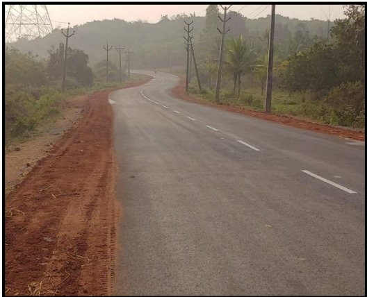
Figure 9: Road condition After FDR
