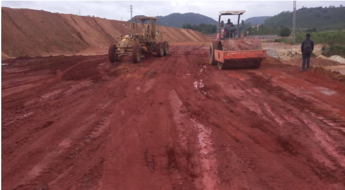
Figure 2: Compaction of the subgrade using a roller
