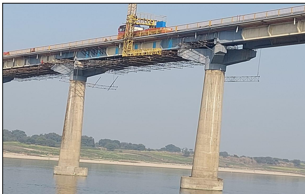
Figure 21: A View of Inspection through Mobile Bridge Inspection Unit of under Rehabilitation Yamuna Bridge at Bendaghat.
