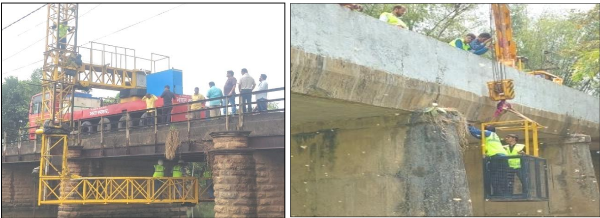
Figure 15: A Typical View of (a) Inspection of Superstructures of HL Bridge over Dhanei River in Budhamba-Buguda road at Chainage 8.988 Km in the Bhananagar Division using MBIU. (b) NDT on the Deck Slab of the Bridge over Local Nalla on Koilama-Brundabanpur Road at Ch-6.200 in Nayagarh(R&B) Division.
