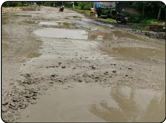
Figure 8: Road condition before FDR
