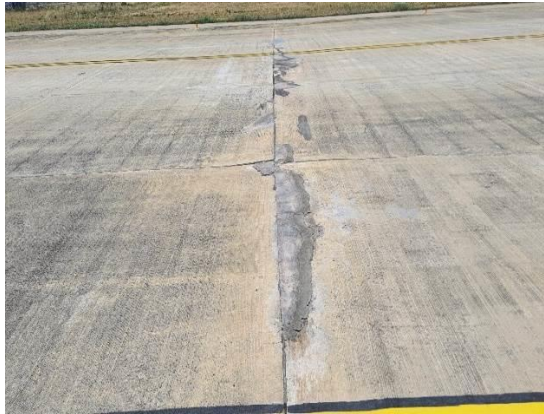
Figure 9: Expansion joint repaired with different repair materials
