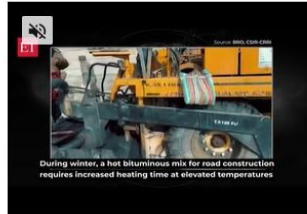
BRO build road under sub-zero temperature at the Indo-China border in Arunachal Pradesh
