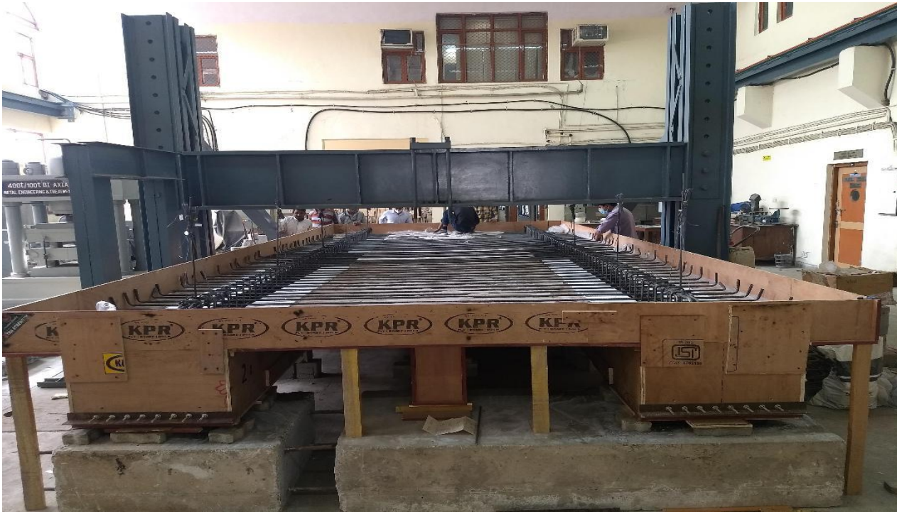
Arc Beam Mould
