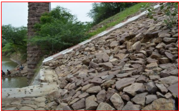
Figure 11: (c) Toe wall is connected with Pier-1
