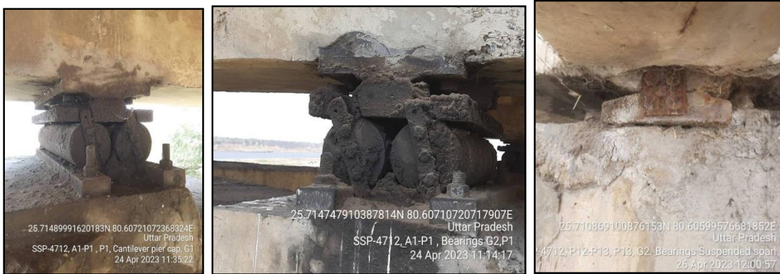
Figure 20: Typical Views of the Temporary Support not Removed on Roller cum Rocker and Rocker Bearings of Yamuna Bridge at Bendaghat.
