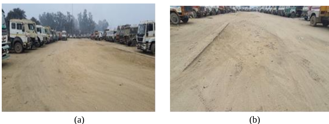
Figure 7: (a) A view of the existing distressed truck parking area used by Multi axle container trucks, (b) A view of the large potholes developed in the existing pavement
