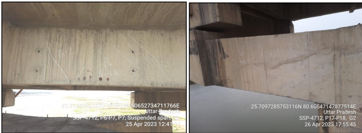
Figure 19: A Typical View of the Crack Observed on Girder G2 in the Suspended Gap Span at Pier P-7 of Yamuna Bridge at Bendaghat. (b) Severe Cracks observed on Cantilever Supporting Bracket below Girder G-2(RHS) at Pier Head of Pier P17 in the Span P17-P18 of Yamuna Bridge at Bendaghat.
