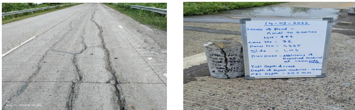
Figure 5: Investigation of distress in PQC, propagation of crack depth to PQC and DLC layer
