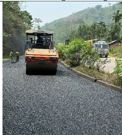
Compaction of Porous layer
