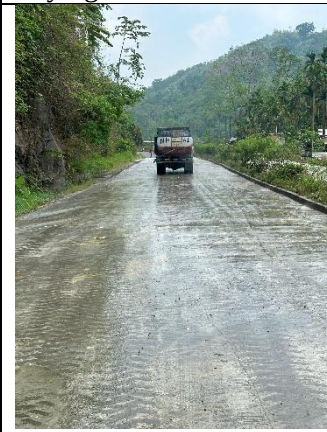
Curing of CGBM layer
