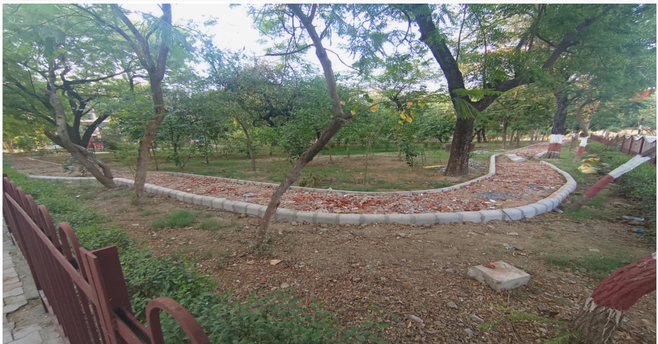
Construction of service road along the Yamuna side Boundary wall, i/c Repair/Plastering from the outer side of the Boundary wall and construction of Walkway/ footpath in the jungle area of Campus -II area along with Peripheral of the lawn area i.e. front of Type -C (33-40) quarters at Campus-I of CRR I Staff Colony, Maharani Bagh, New Delhi-110065.
