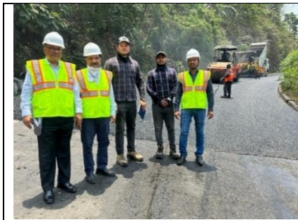
Laying of Porous Bit. Layer May 2024
