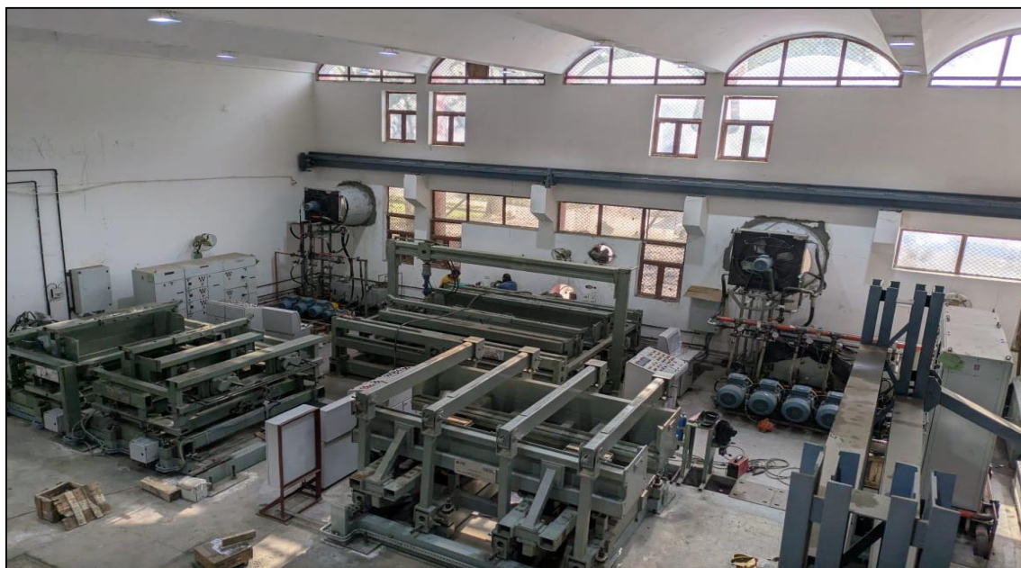
Figure 3: View of Installed three rigs of the Test facility at CRRI
