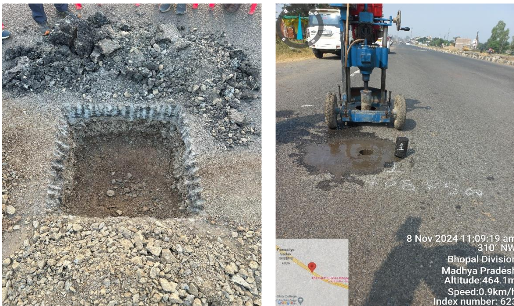
Typical view of testing under progress on the project road.
