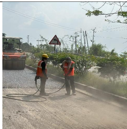
Surface Cleaning /Brooming
