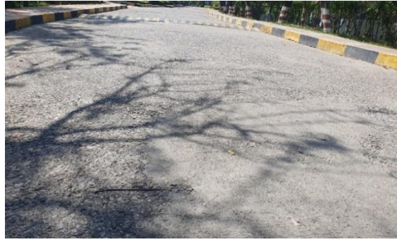
Fig 14: A typical ravelled surface repaired with cement mortar
