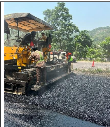
Laying of Porous Bit Mix
