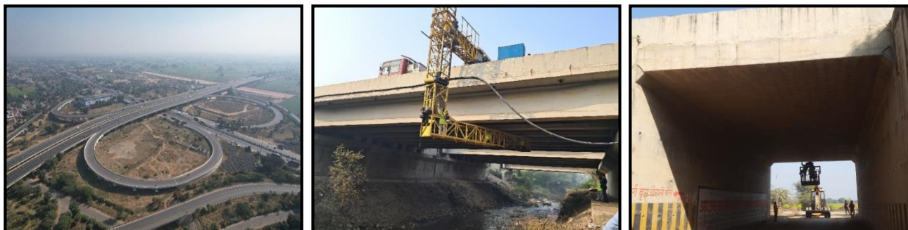
Figure 8: Different structures of Yamuna Expressway and the means of their visual inspection
