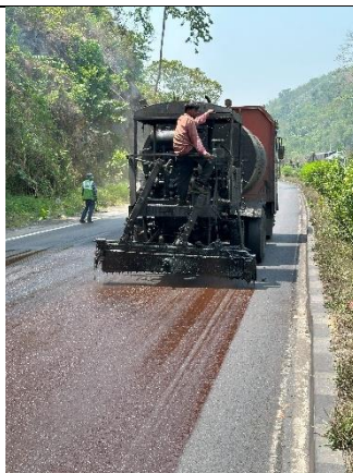
Tack coat Application
