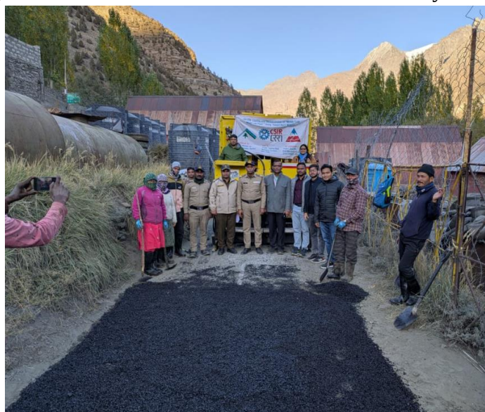
View of laid section using Tunnel Muck at Istingira, Lahaul & Spiti, Himachal Pradesh
