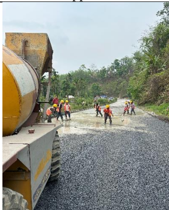
Grouting on Porous Bit. Layer
