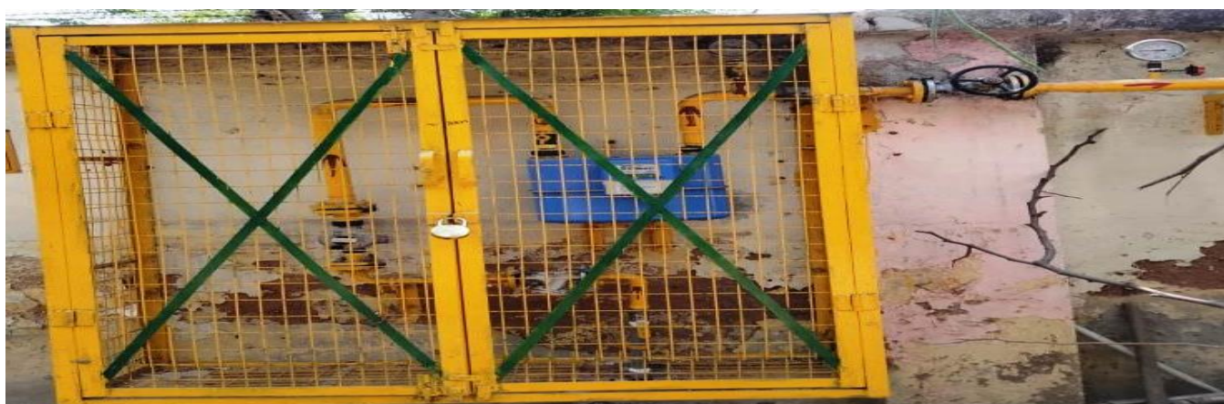
Supplying Installation Testing & Commissioning of Dual Fuel Kit in Existing 125 kVA & 40 kVA DG Set Installed at CRR I Staff Colony Maharani Bagh N.Delhi-110065
