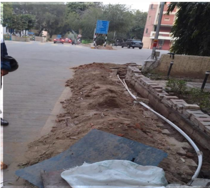
Providing and laying pipeline network for potable water at CRR I Staff Colony, Maharani Bagh, New Delhi-110065
