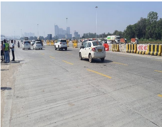
Photo 30: A view of the Dwarka Expressway Toll Plaza (KM 8.700 to 9.500 KM)
