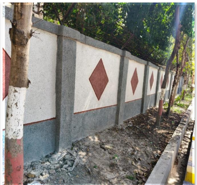
Repair & Face Lifting of Boundary Wall with Grit Wash at CRR I Staff Colony, Maharani Bagh New Delhi - 110065
