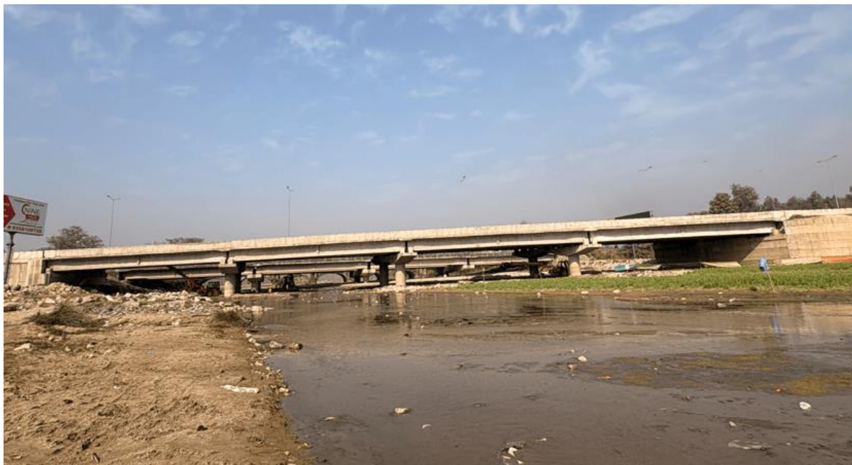
Photo 5: View of Major bridge at Ch.34+728
