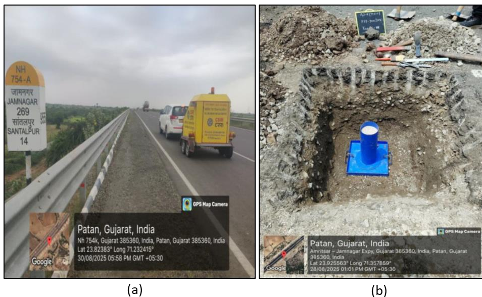
Photo 17: (a) Falling Weight Deflectometer (FWD) survey (b) Sand replacement test to determine densities within test pit
