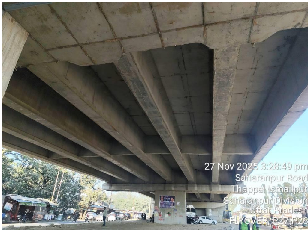
Photo 4: View of Elevated bridge at Ch.36+415
