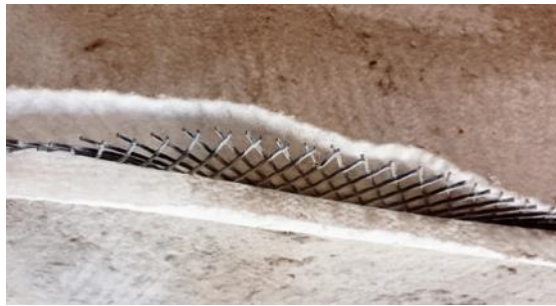
Photo 27: Typical photo of geocomposites
