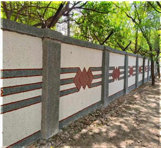
Repair & Face Lifting of Boundary Wall with Grit Wash at CRR I Staff Colony, Maharani Bagh New Delhi - 110065
