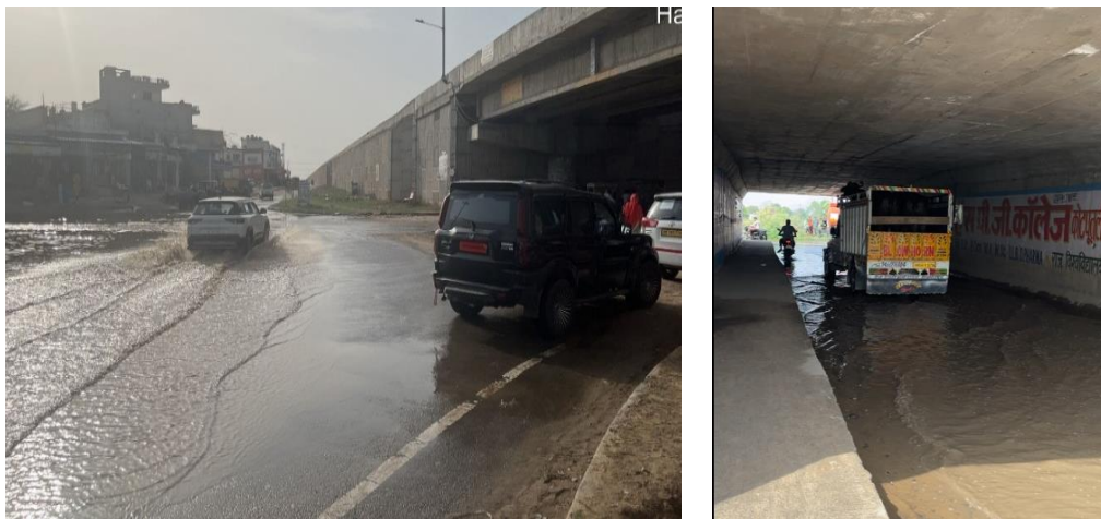
Photo 13: Waterlogging in Highway Underpasses
