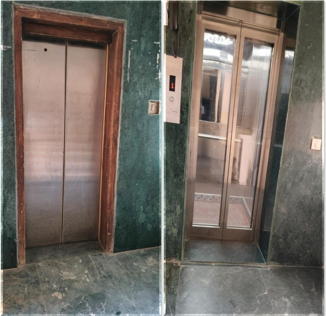
Supplying, Installation, Testing & Commissioning of New Lift in Phase-I MS Building at CRR I Staff Colony, Maharani Bagh New Delhi - 110065
