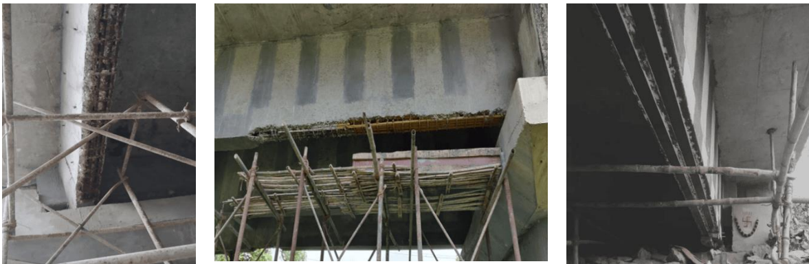
Photo 1: Strengthening of Corroded Bridge Girder using CFRP Composites
