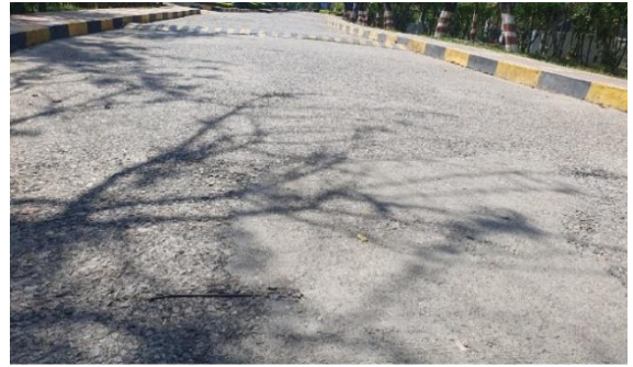
Photo 33: A typical ravelled surface repaired with cement mortar
