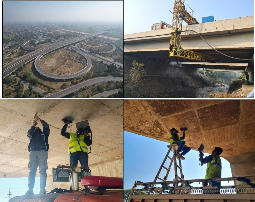
Photo 3: Different structures of Yamuna Expressway and the means of their NDT
