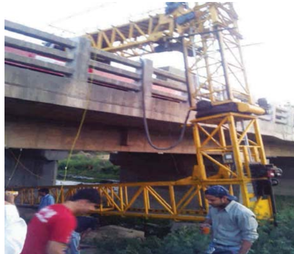
Figure 5 : MBIU under Operation on a Bridge on NH24
