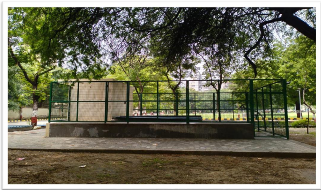
Construction of Under Ground Water Tank for STP Treated Water at CRR I Staff Colony, Maharani Bagh, New Delhi-110065
