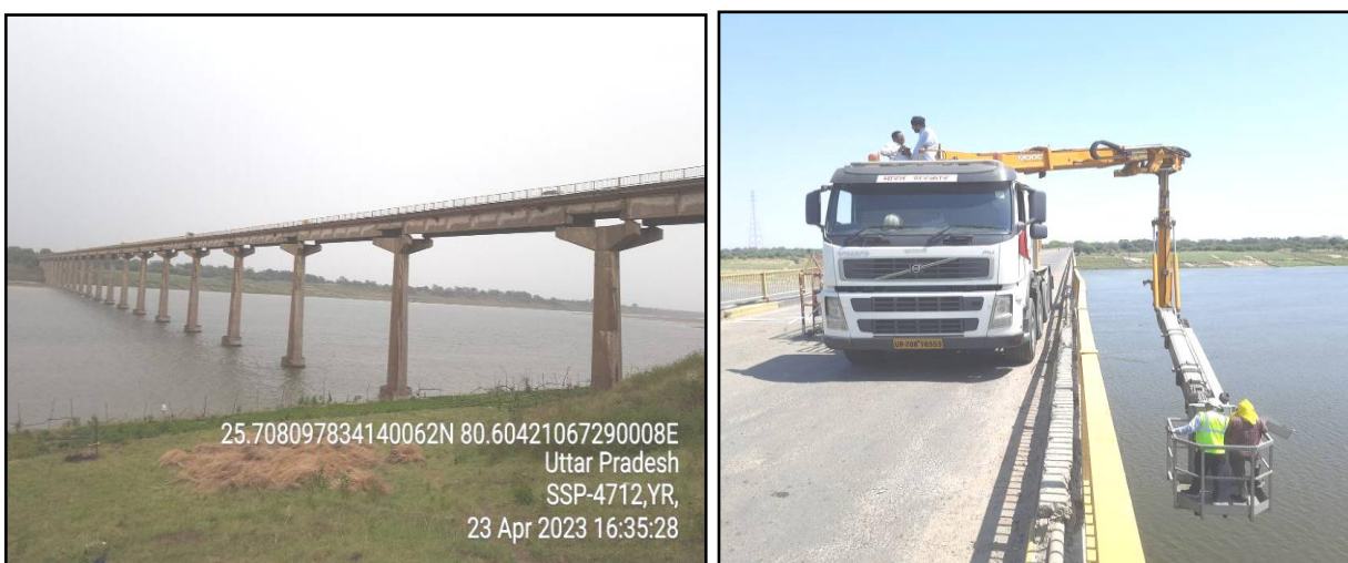
Figure 17: General View of Span Arrangement of Yamuna Bridge at Bendaghat and Inspection through Mobile Bridge Unit of Yamuna Bridge at Bendaghat.
