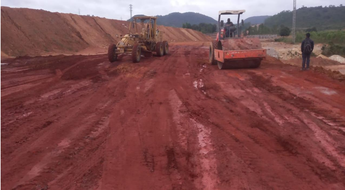
Figure 2: Compaction of the subgrade using a roller
