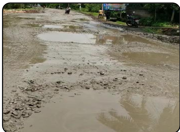
Figure 8: Road condition before FDR
