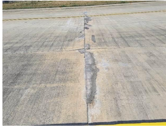
Figure 9: Expansion joint repaired with different repair materials
