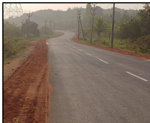
Figure 9: Road condition After FDR
