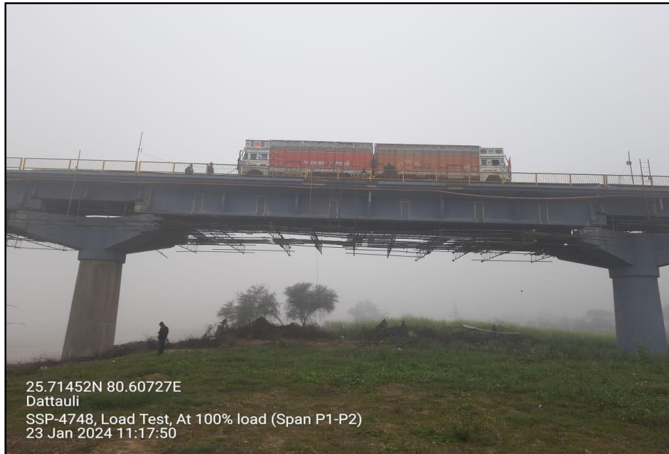
Figure 22: A Typical View of Load Test on Span P1-P2 of Yamuna Bridge at Bendaghat.
