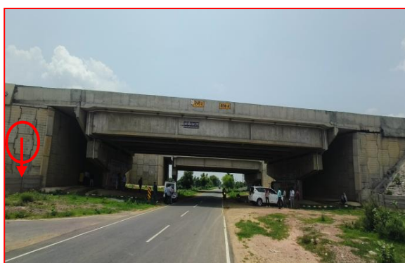
Figure 4:(a) Intersection of SH at Km 137+300 on Vadodra–Delhi Expressway
