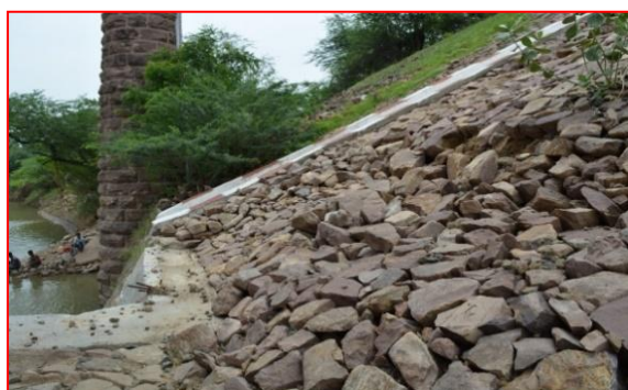
Figure 11: (c) Toe wall is connected with Pier-1
