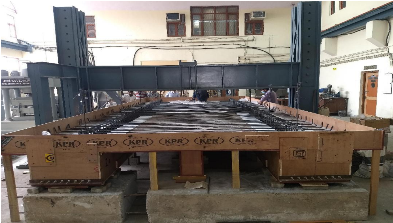
Arc Beam Mould
