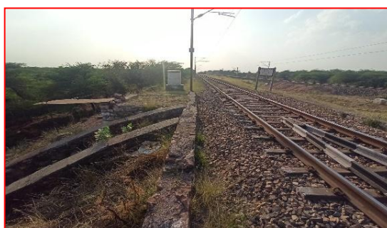
Figure 11: (b) The approach to Abutment-1 is constructed on 13.5m high embankment
