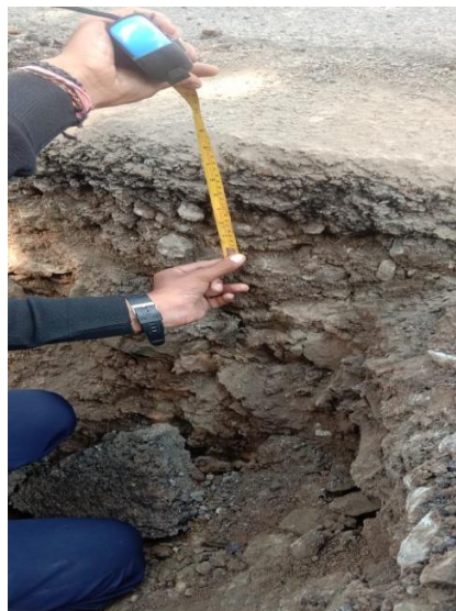
Figure 4: Thickness measurement of the existing bituminous road crust layers in progress
