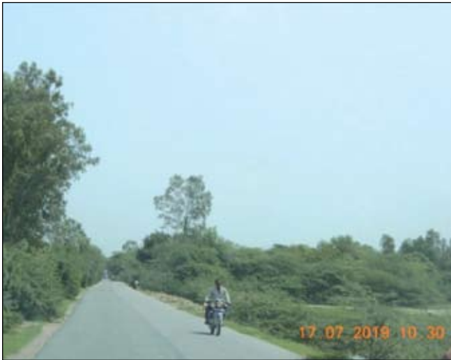
Absence of 'Curve Ahead', 'Chevron Signs' and protruding trees obstructing the sight distance
