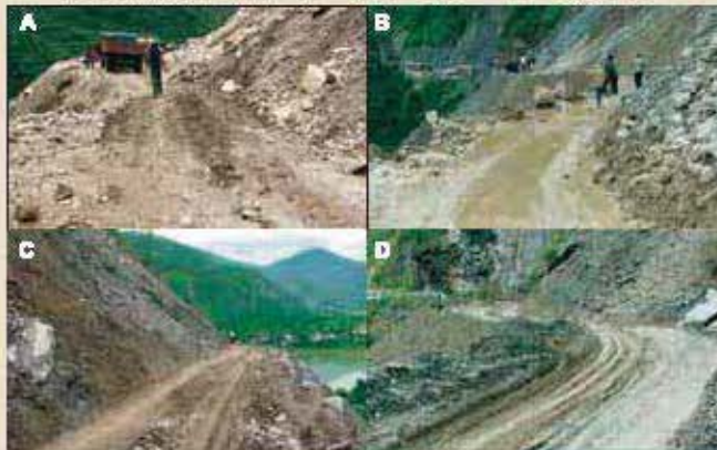
Fig 2: Breached roads at different places (from Chomoli to Gangotri), caused by failure of overburden and varied size of boulders
