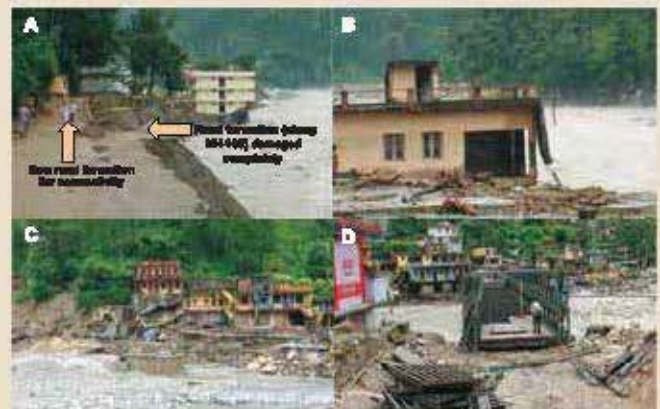
Fig 3: Road formation washed away through floods (A), Houses and Bridge destroyed at Gangotri (B & C), Bridge construction work is under progress at Gangotri (D).
